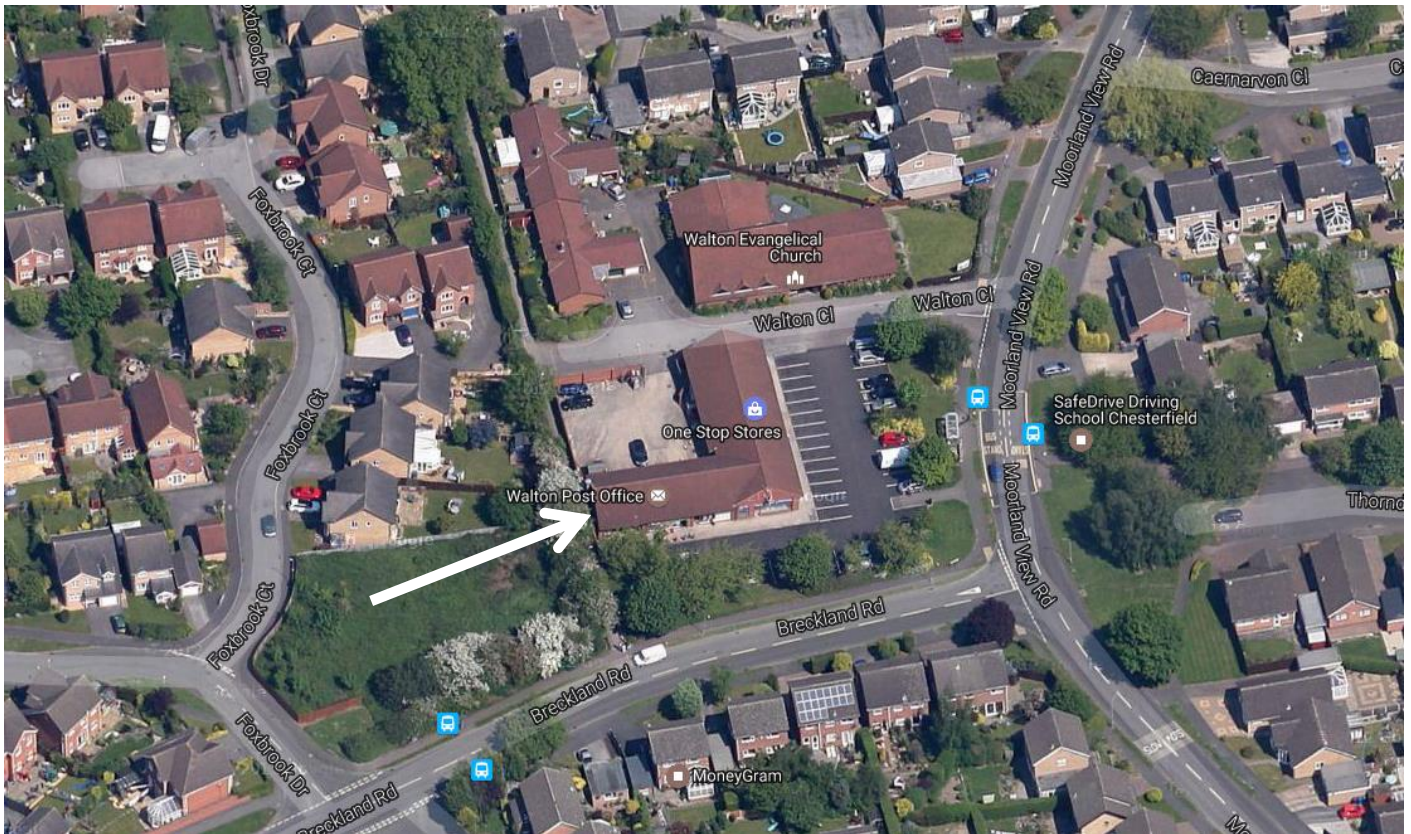
Figure #2 – aerial view of the premises.
